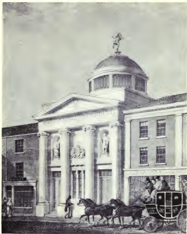
THE NEW COMMERCIAL BUILDINGS AND POST OFFICE
